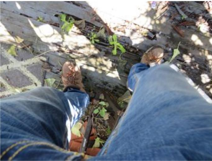
Deck is broken/damaged. Replacement required
