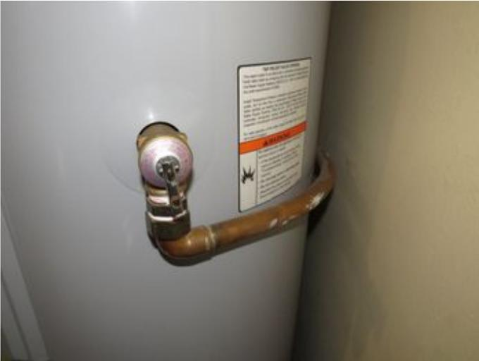
The water heater is equipped with a mandated pressure-temperature relief valve.
