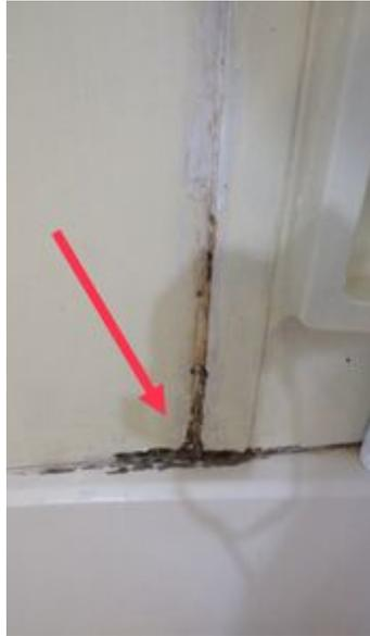
The tub/shower drains too slowly, caulk missing in several areas and should be serviced, because such blockages can progress beyond the drain trap and involve the main waste line.
