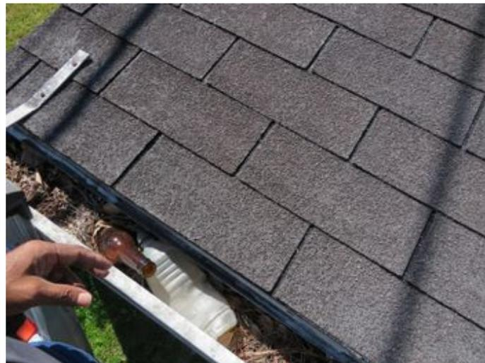
Gutter is missing in the indicated area. Repair recommended
