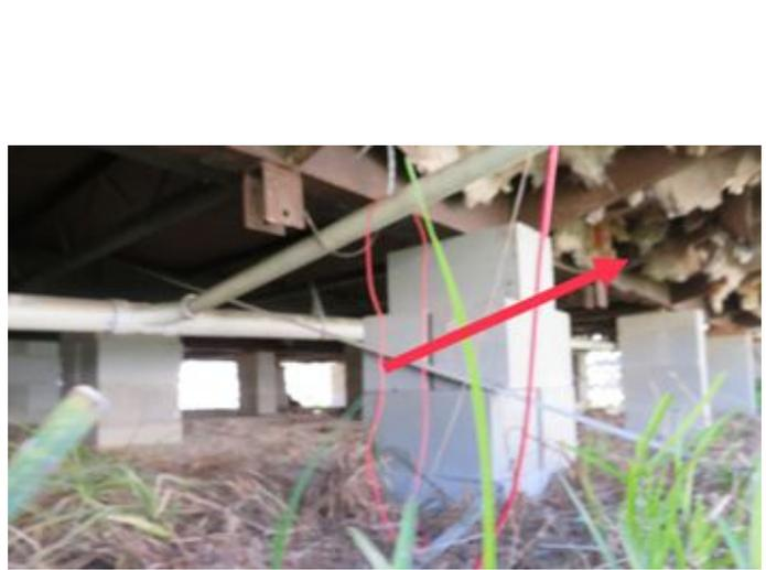
Indicated (broken /missing vapor barrier)area needs to be repaired
