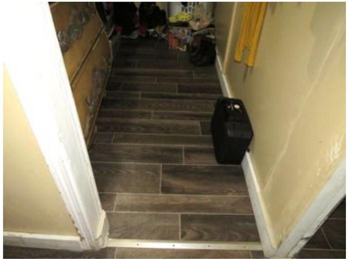
Indicated area needs to be repaired (transition strip missing by the door on the floor, cracks on tiles). Repair required
