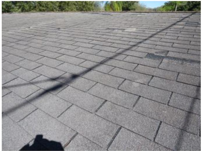
Overall condition of the roof appears to be in unsatisfactory (excessive granular loss, brittleness, missing shingles) condition. Replacement/further evaluation recommended
