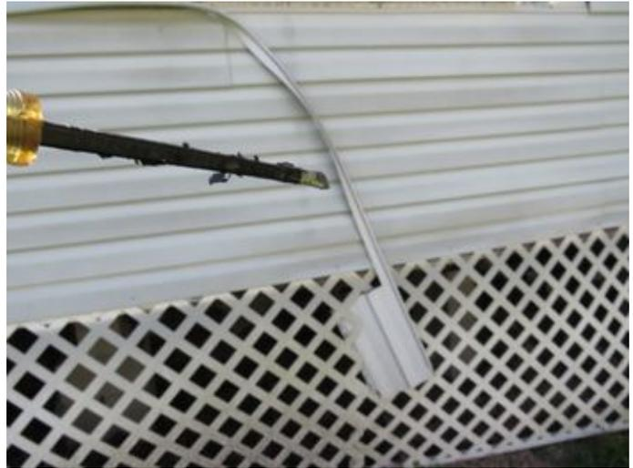
The house walls finished with vinyl siding. Indicated areas observed minor cracks. Repair recommended
