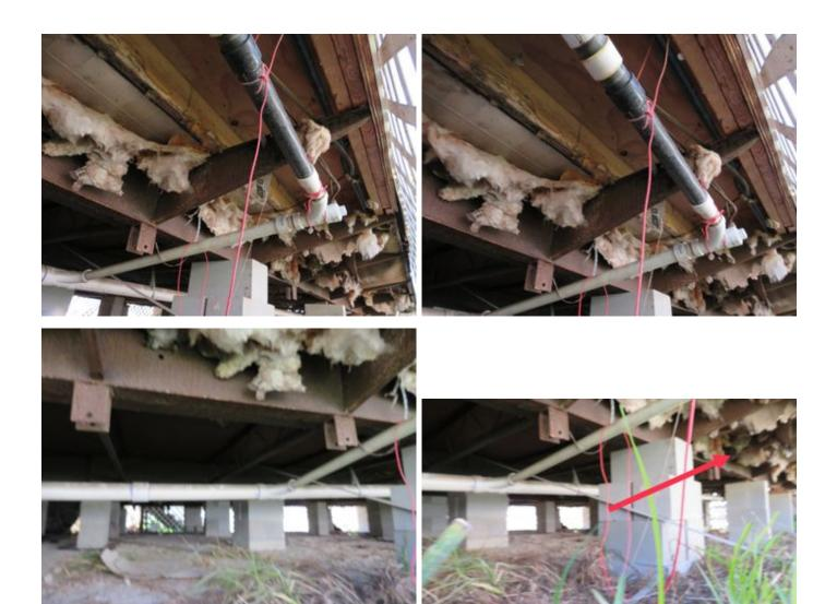
Indicated (broken /missing vapor barrier) area needs to be repaired
