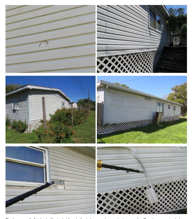
The house walls finished with vinyl siding. Indicated areas observed minor cracks. Repair recommended
