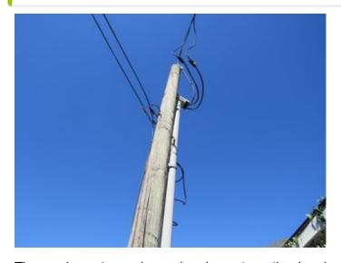
The service entrance is overhead, mast weather head, and cleat are in acceptable condition.
