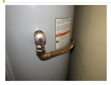
The water heater is equipped with a mandated pressure-temperature relief valve.
