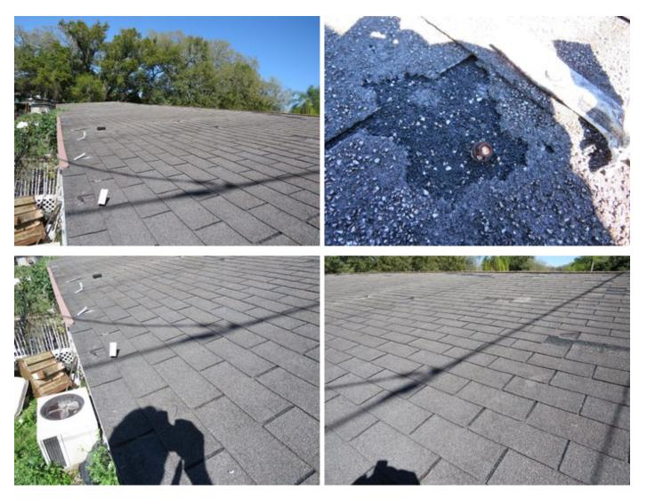
Overall condition of the roof appears to be in unsatisfactory (excessive granular loss, brittleness, missing shingles) condition. Replacement/further evaluation recommended
