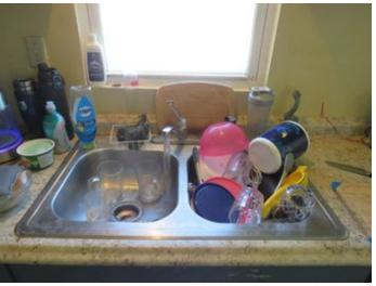
Appears to be in satisfactory condition. However deficiencies observed (leaks on the faucet, defective spray wand, peeling off pieces from underneath the sink ) in the indicated area . Repair recommended
