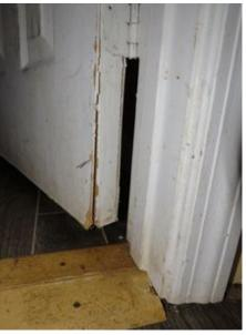
Door found in unsatisfactory condition. And windows are difficult to operate. Repair/replacement required
