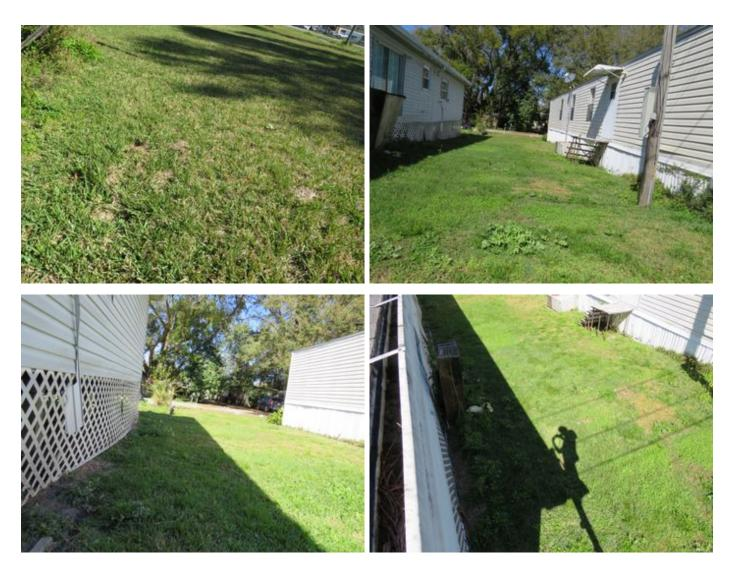
The residence is situated on a flat level pad, which would typically not need a geological evaluation. However, we do not have the authority of a geologist and you may wish to have a site evaluation. Due to the rain/other causes, some soil washed away/missing from the indicated areas. Sand/soil fill recommended
